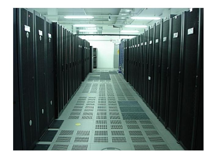
SGI UltraViolet with air guides in front to improve cooling efficiency (2012)
